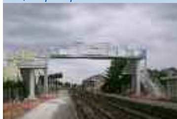
Passerelle SNCF Rang-du-Fliers
