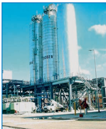
Structure support de silo.
